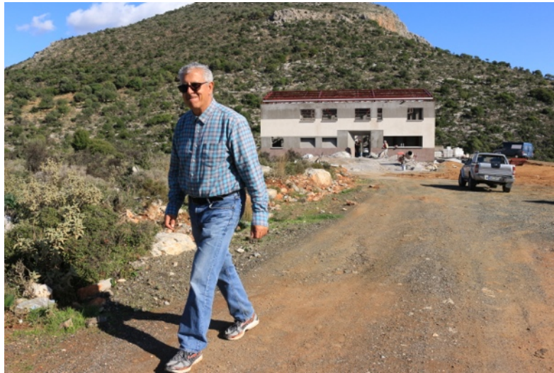
Tsimpidis in the driveway of his new winery, still under construction.
